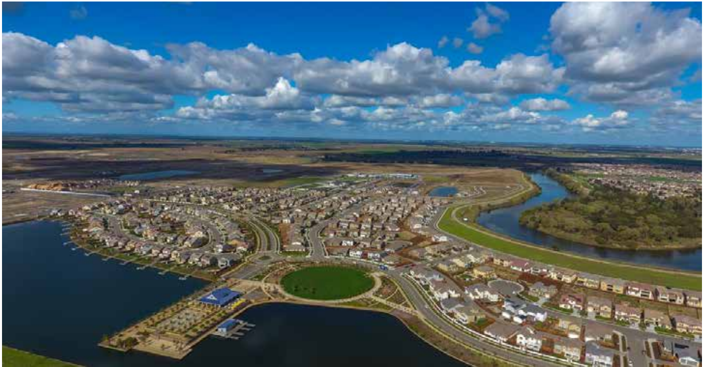
Phase 1 of the River Islands development in Lathrop, California
